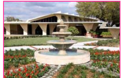
The organic design that graces the campus of Florida Southern College is the work of Frank Lloyd Wright.
